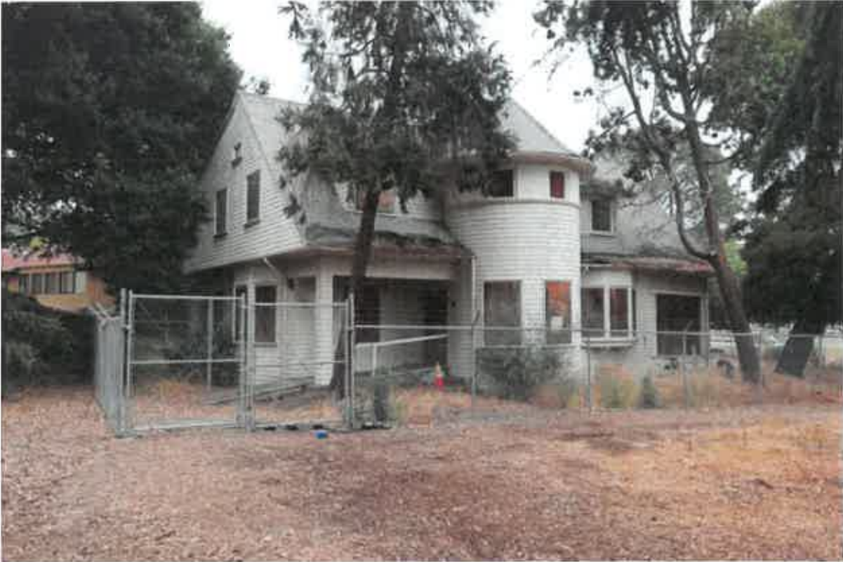
Fig.3 – Superintendent's Residence/Whitecotton Cottage, West side, 2018
