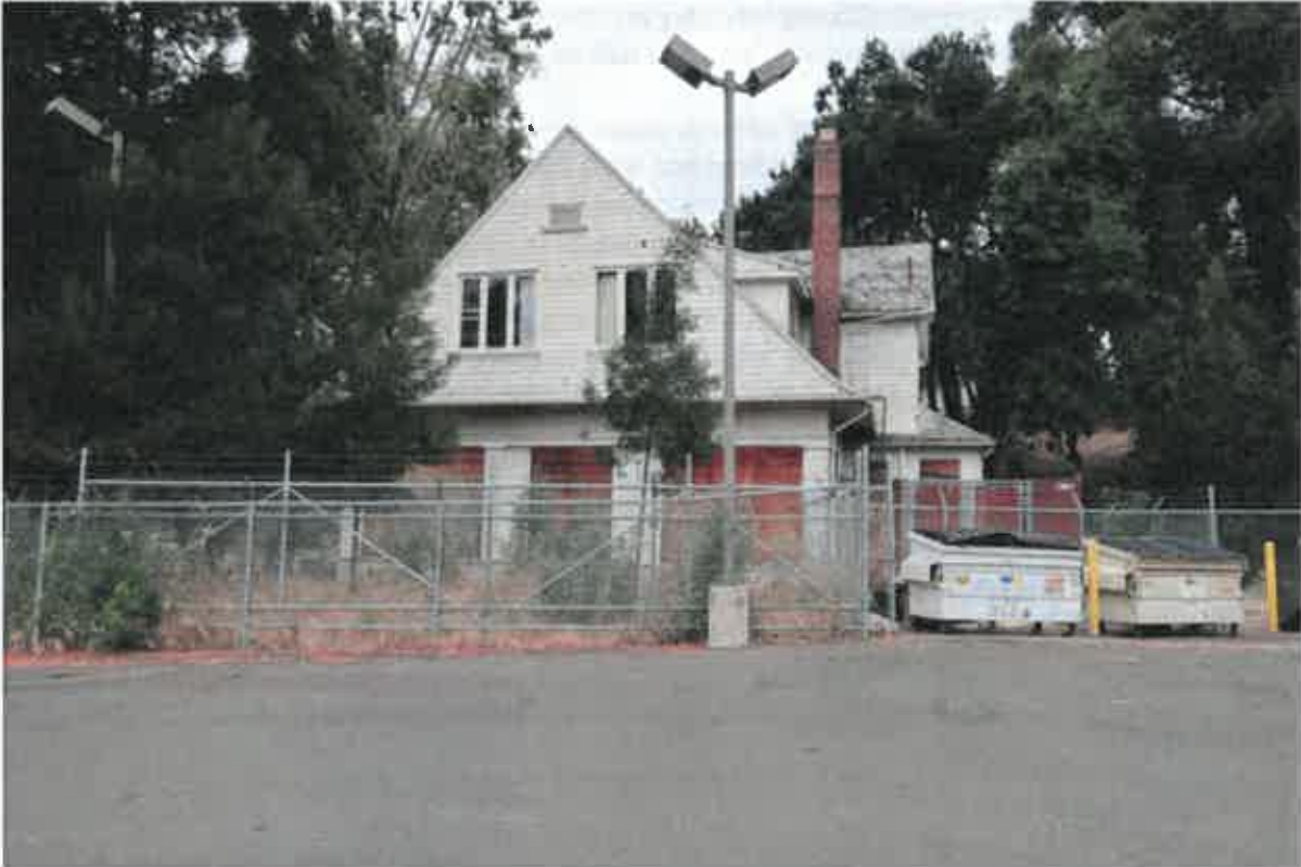
Fig.1 – Superintendent's Residence/Whitecotton Cottage, Front (south), 2018
